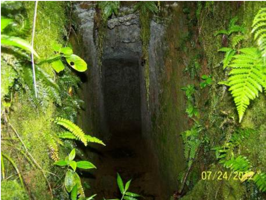
Tunnel in the upper Olum watershed, constructed by the Japanese in World War II.
