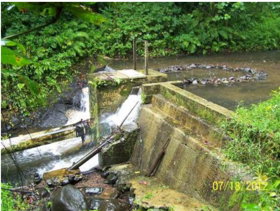
Water supply reservoir on the Olum stream, near the proposed protection area, Olum watershed
